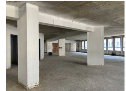
Fig. 16: Current interior view of a typical floor level, showing how much space is taken up by the central core and awkwardly-placed structural columns, reducing the useable floor area. Photograph by the author.
