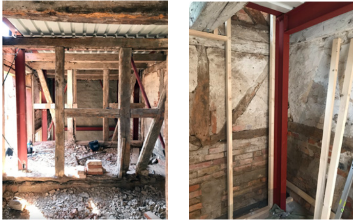
Construction site images showing the new metal structure next to the existing one. Image: Author, 2022
