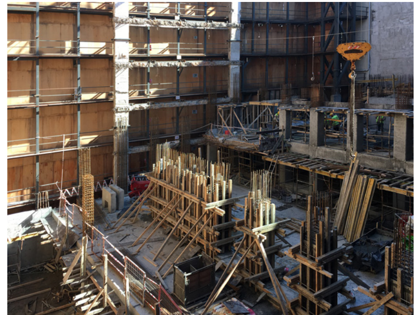
Photographs from the construction: Preservation, demolition and construction, all at once.
