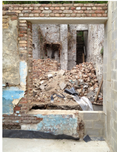
Fig. 11: Bricks reclaimed and hand-cleaned on site, then used to repair damaged sections of the existing outbuildings. Courtesy of Simon Pirlot Architecte.
