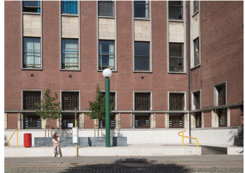
Intervention at entrance area - RE-ST, picture by Stijn Bollaert, 2019
