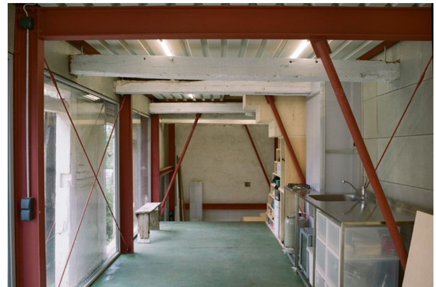
Interior showing the ground floor of the workshop with a floor sunflower-oil pigmented lime screed on an insulation made from recycled glass. Image: Zara Pfeifer, 2023
