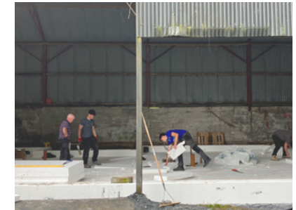
Image 22: Existing shed shown in context Image 23: Existing shed interior Image 24: Excavation of shed floor to required levels Image 25: Preparation of compacted hardcore and sand blinding Image 26: Setting out of raft slab relative to existing shed Image 27: Installation of EPS insulation formwork Image 28: Reinforcement mesh ahead of concrete pour.
