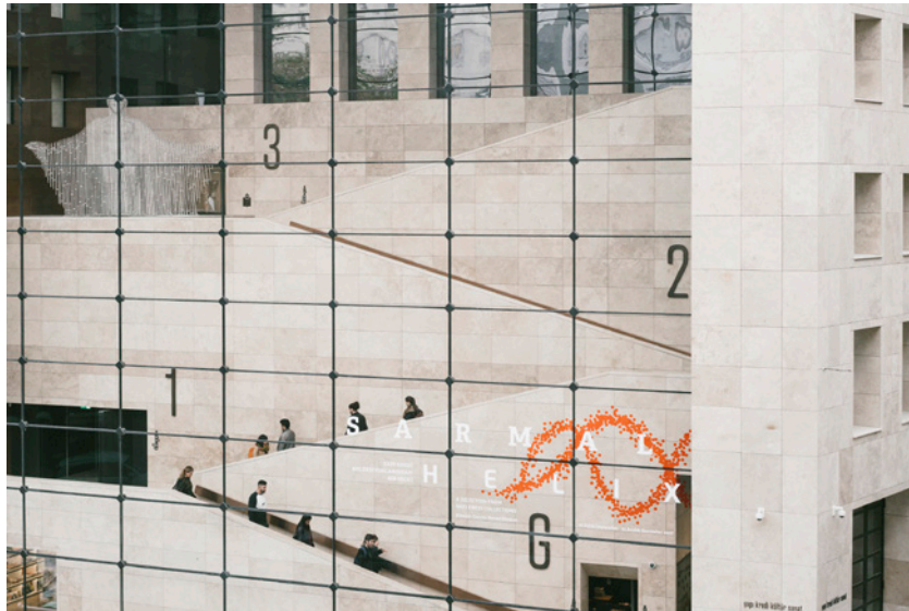
The emergent space (atrium) at the front became the confrontation area of both the old and new building with the city. Photograph: Ekin Özbiçer
