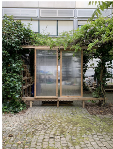
Strategy 3. Displacing elements, transforming their original meaning : Reusing the polycarbonate panels used as envelopes for a greenhouse for creating mobile demarcations within a courtyard, 2 nd and 3 rd editions - 2022-2023. © Camille Fauvel and students documentation
