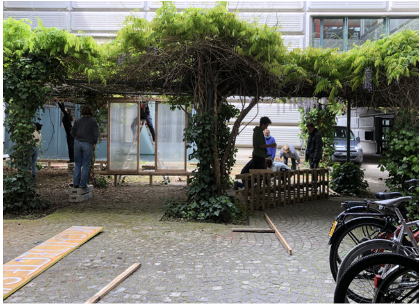
Subtraction of elements used as part of a greenhouse in Evian and reused as panels and sits for a public space on the EPFL site. © Camille Fauvel (2022)
