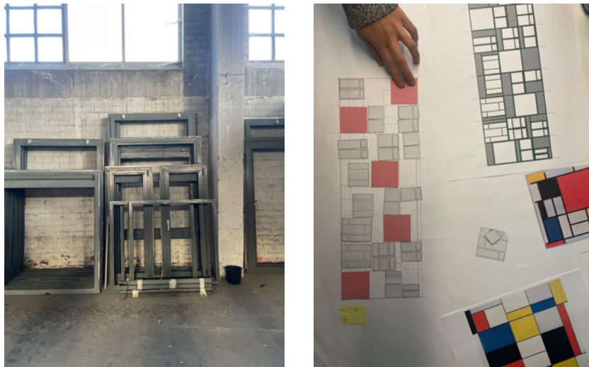
The steel window frames being reclaimed from a nearby demolition site in Mechelen. Storage of the window frames and design exercise for positioning of the reclaimed frames in the front façade.
