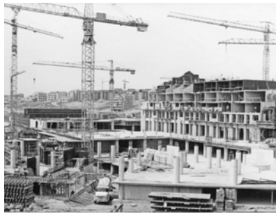
Fig. 20: Archive photo showing the construction of Louvain-la-Neuve on the concrete slab or dalle . Source: Archives de l'Université catholique de Louvain.
