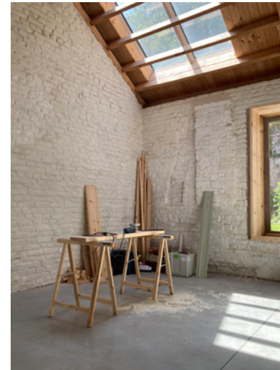
Fig. 9: Interior of the former gunsmith's atelier during renovation into a maisonnette. Photograph by the author.
