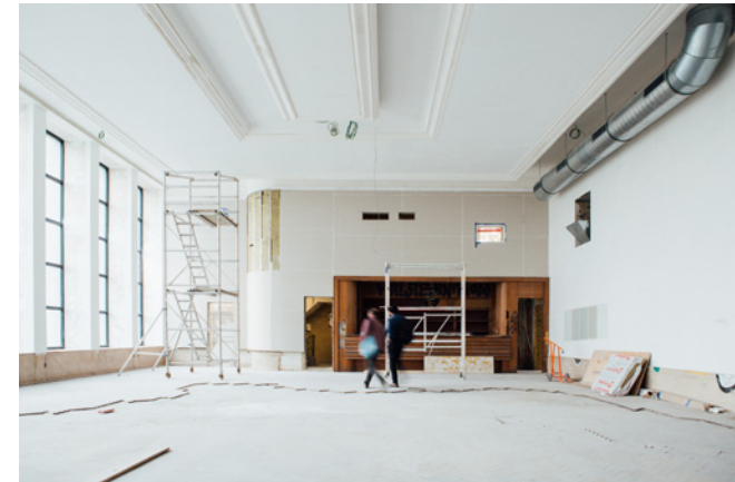
In the second room, the original parquet flooring is carefully dismantled, repaired, treated, and reinstalled to preserve the ambience and history of the place. The same applies to the bar.
