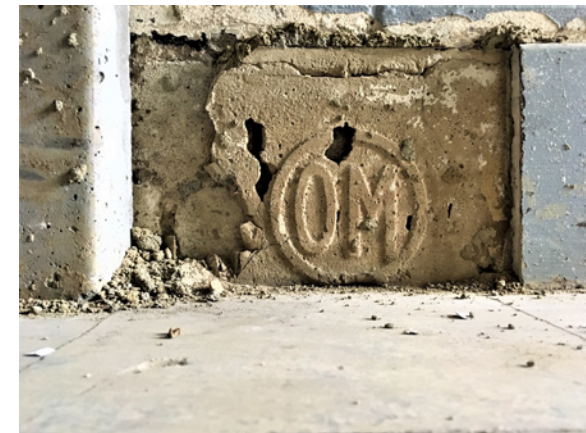
Imprint left by the dismantling of a glazed ceramic. The study and dismantling of the building highlighted the unique, local character of the original construction.
