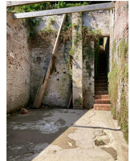
Fig. 10: New exterior courtyard created by removing the dilapidated roof of the former stable. Photograph by the author.
