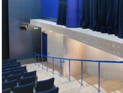
Fig. 23: Interior of the new theatre hall, showing the tiered seating and steps extending below the cut-through and polished edge of the former ground floor plate and concrete dalle structure. Photo by the author.
