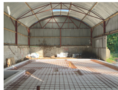
Image 22: Existing shed shown in context Image 23: Existing shed interior Image 24: Excavation of shed floor to required levels Image 25: Preparation of compacted hardcore and sand blinding Image 26: Setting out of raft slab relative to existing shed Image 27: Installation of EPS insulation formwork Image 28: Reinforcement mesh ahead of concrete pour.
