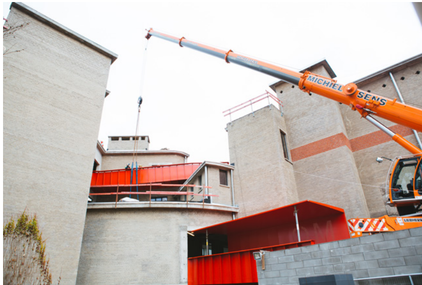
Installation of the upper walkway, linking the office areas to the new roof terrace.
