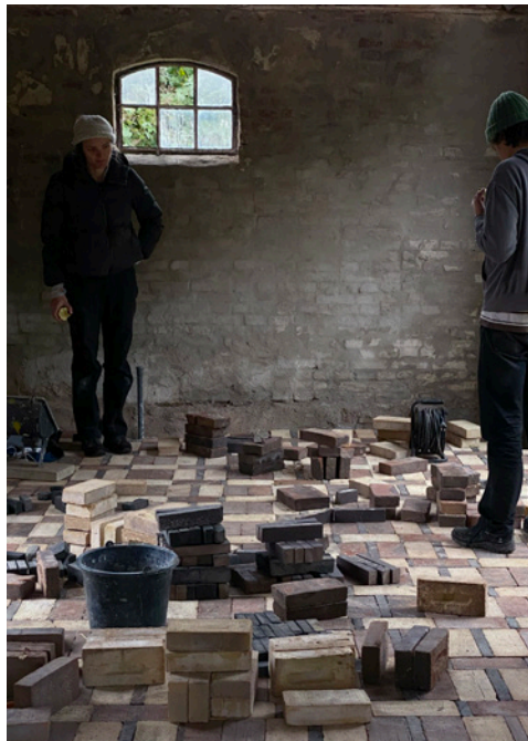
The Case 1 project explores the interplay between reusing salvaged materials and valuing the existing architecture. The flooring is made from leftover bricks from a nearby factory, gruppe-aja
