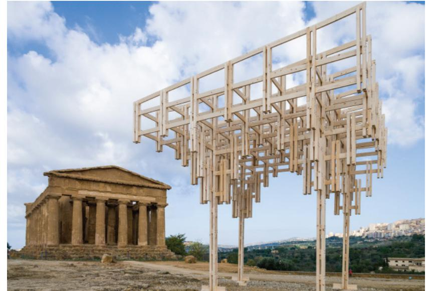
Conceived during a workshop held in 2013 in the Archaeological Park of Agrigento, this pavilion explored the design and construction of lightweight, temporary structures to shelter archaeological excavation works otherwise exposed to the weather. The traditional bracketing system was reinterpreted in the design, yet, it keeps an essentiality both structurally and aesthetically, and present an intrinsic elasticity, which lessens the impact of lateral forces by acting as a shock absorber.
