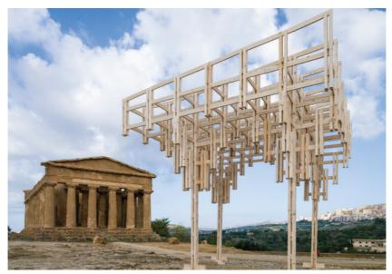
Conceived during a workshop held in 2013 in the Archaeological Park of Agrigento, this pavilion explored the design and construction of lightweight, temporary structures to shelter archaeological excavation works otherwise exposed to the weather. The traditional bracketing system was reinterpreted in the design, yet, it keeps an essentiality both structurally and aesthetically, and present an intrinsic elasticity, which lessens the impact of lateral forces by acting as a shock absorber.
