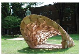
The external surface of the pavilion is a smooth continuous curve while its internal surface is irregular due to the different depths of the triangular units. These units posed a challenge in terms of connections to each other due to their wide range of angles; finger joints resolved the issue by increasing the contact surface area.
