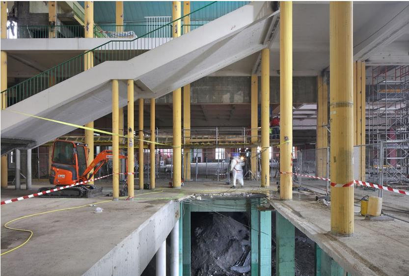
New railings and steel reinforcements superimposed onto the existing, 2021, ©Filip Dujardin
