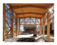
The overall concept alternated between green spaces, fountains (used for aquaculture) and paths, and was inspired by a network of traces from old nautical charts of Polynesia and the Marshall Islands. The CLT structure of this ephemeral building was designed to be easily dismantled after the Expo and reused elsewhere.
