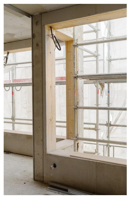
Fig. 2 - The hempcrete is the whole envelop of the building. The insolation is the whole wall.
