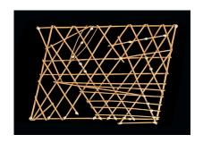
Sea and island temporary pavilion for Milan EXPO 2015. The hanging structure is realised in bamboo and the structure is built in CLT posts, beams and panels. The pavilion was deconstructed and used afterwards for another project.
