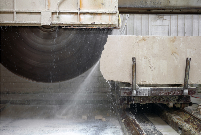
Fig. 6 - Through one economical gesture, the cut, the fragment becomes element of architecture.
