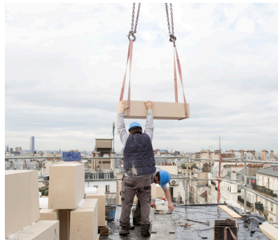
Fig. 4 - The stones are being assembled on the site. They bear the traces of their belonging to the ground.
